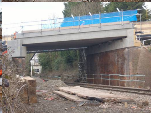
Main Structure In Place
