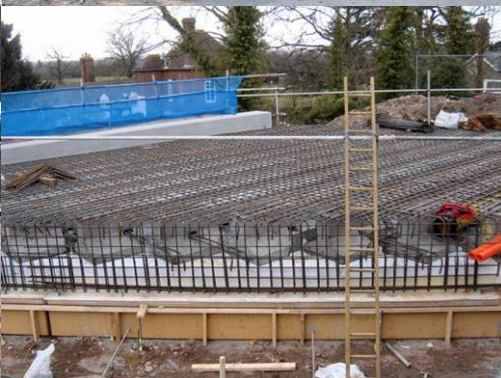
Concrete Girders For Road Bed
