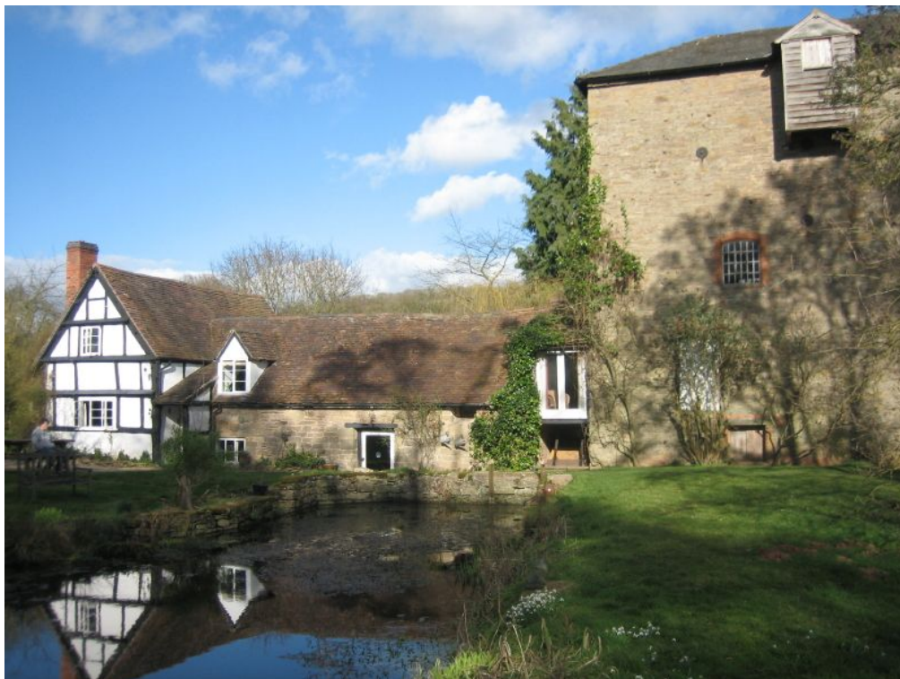
Beanhouse Mill is a late 19th century watermill and one of the last to be built in Herefordshire. It is also known as Archer's Mill, after one of the early millers. The mill was last used for milling in the 1960's or 70's.
